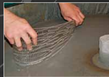
Taglio e sagomatura. Cutting and shaping on each panel.
